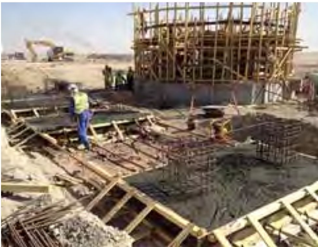
CPF – Hot Oil Heater Foundation; Hot Oil Heater Pipe Rack Foundations
