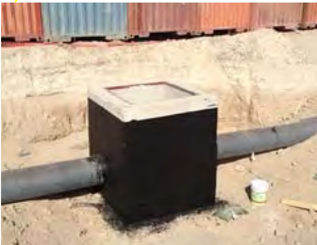
CPF – Various Catch Pits and Underground Piping for Storm Water
