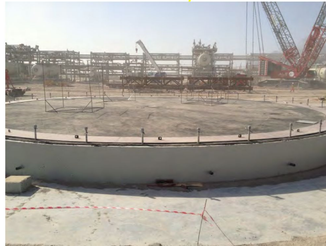
CPF – Wash Water Tank Base; Potable Water Tank Installed; Raw Water Tank Base; Produced Water Tank Base; Buffer Tank Base
