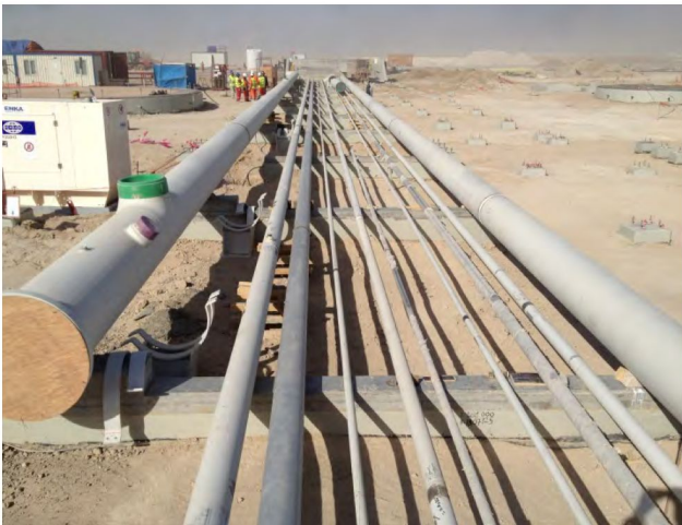
CPF – Piping Installation on Sleepers and in Piperacks
